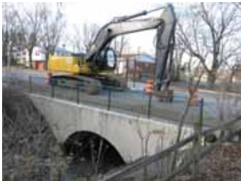
Before and after photos of the Arcadia Boulevard Bridge Replacement Project that replaced a 50 year old under-capacity metal culvert with a new, concrete box culvert.
