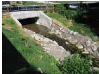
Before and after photos of the Arcadia Boulevard Bridge Replacement Project that replaced a 50 year old under-capacity metal culvert with a new, concrete box culvert.
